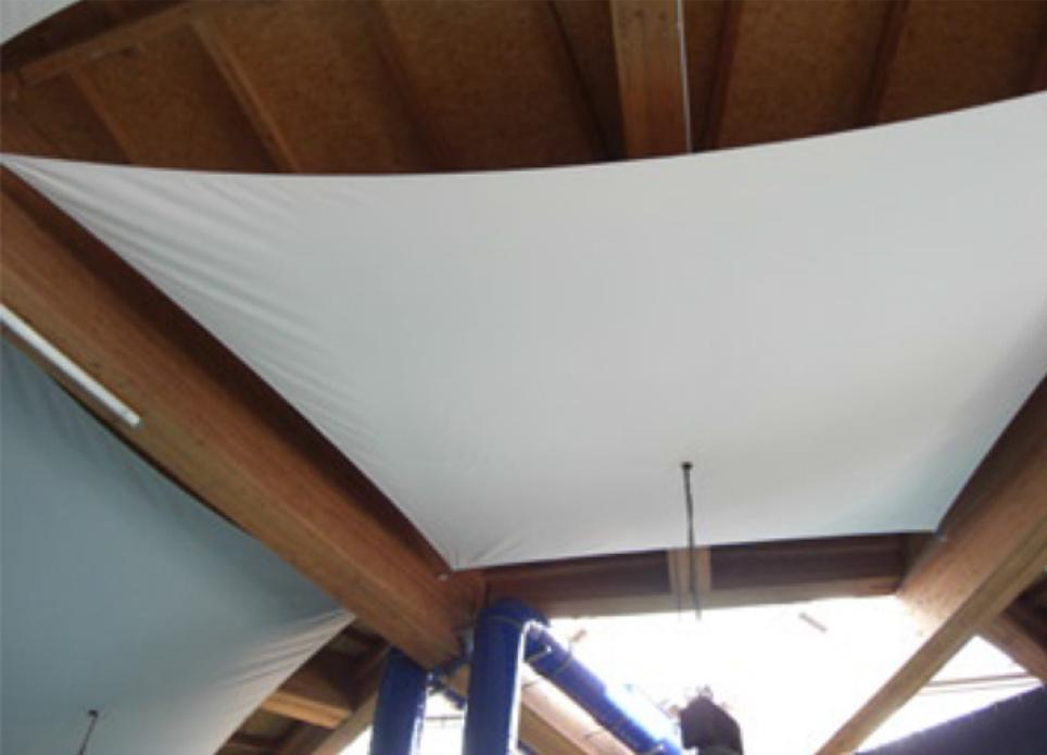
THE ACOUSTIC SAILS ARE RESISTANT TO CHLORINE CORROSION, AND ALSO IMPROVE THE ACOUSTICS OF THE BUILDING.
