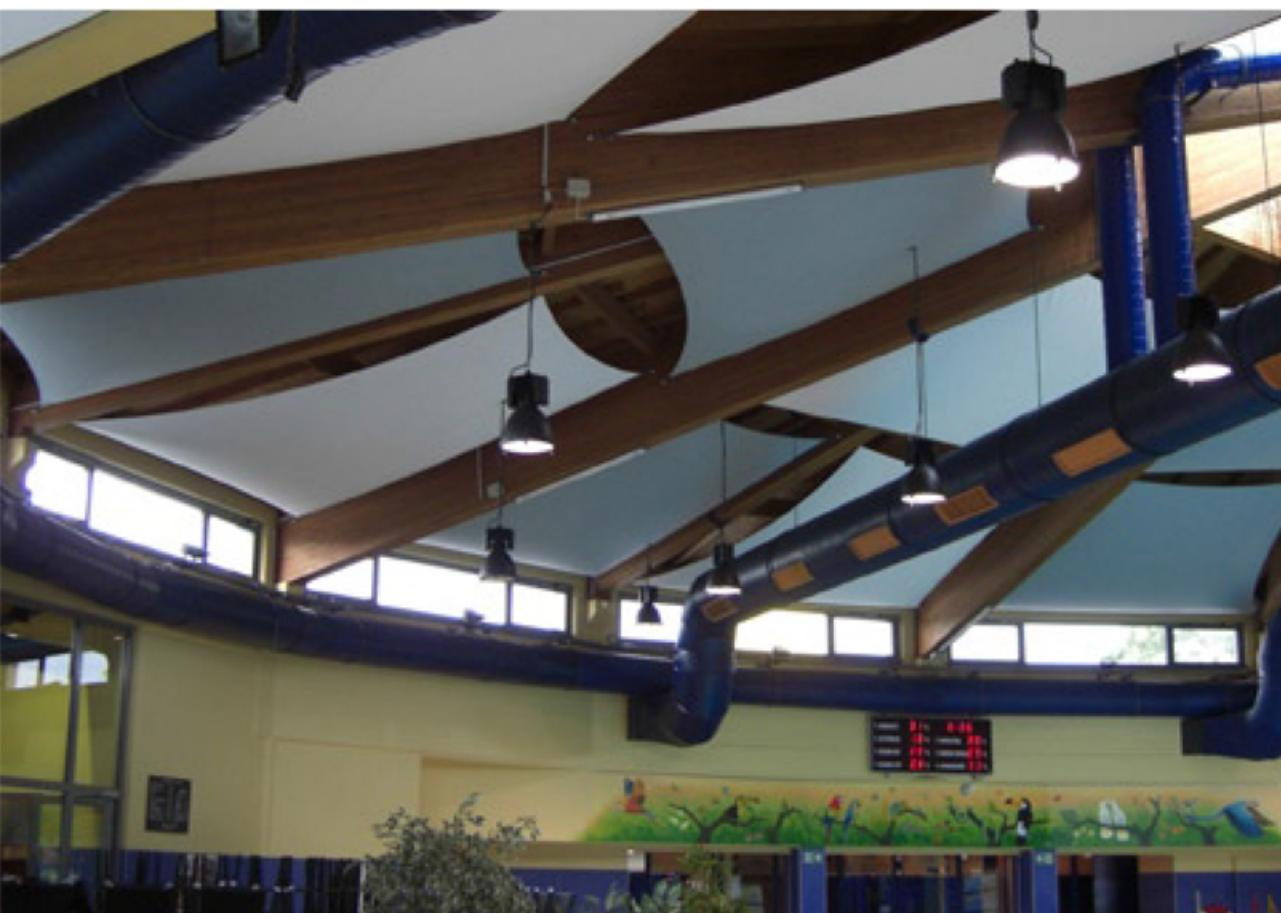
**PLANEX TECHNIK IN TEXTILE GMBH** took charge of a project to renovate an indoor swimming pool, using sails inside the building for better noise absorption and to improve the acoustics of the hall, while adapting to its interior design.
